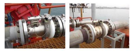
Shown is a Dual release ERC incorporating both a Cable and Hydraulic Release.
